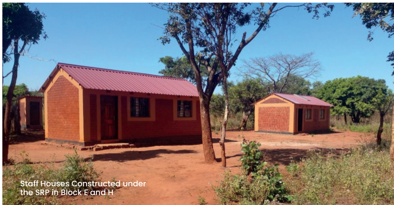
Figure 2.40: Staff Houses Constructed under the SRP in Block E and H
