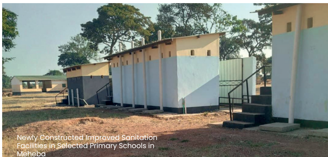
Figure 2.31: Newly Constructed Improved Sanitation Facilities in Selected Primary Schools in Meheba
