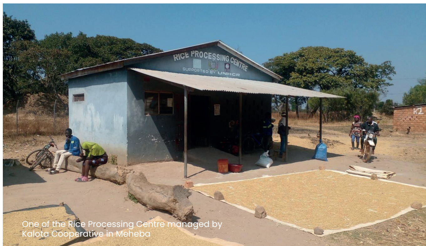
Figure 2.54: One of the Rice Processing Centre managed by Kalota Cooperative in Meheba
